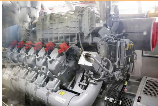
Installation of a 1.3MW CHP system and a Flu-Ace heat recovery system
